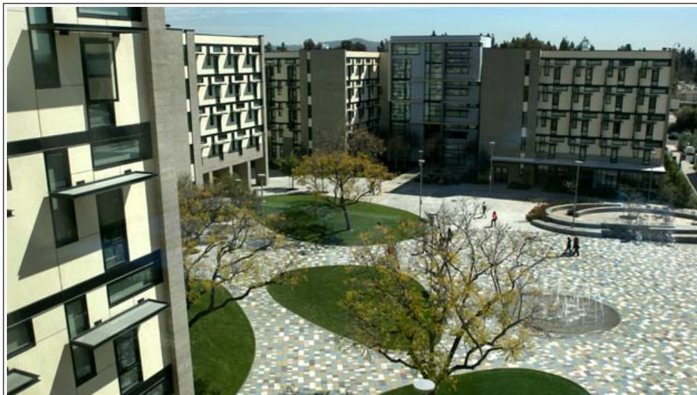
Energy-efficient windows with sunscreens are one of the features that won the new student housing Platinum (LEED) certification by the U.S. Green Building Council. Photos: Karen Tapia Download Image
